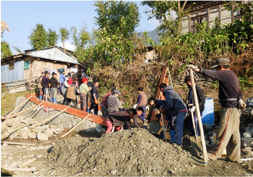
Pic 7. Picture of footpath construction here
